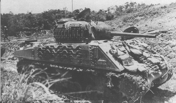
A Marine M4A2 (W) medium tank of the 1st Marine Tank Battalion on Okinawa. This is one of the late production types with the new commander's all round vision cupola. This unit painted its tactical insignia on the upper edge of the turret due to the use of extensive track blocks, in this case a circled number 1.
