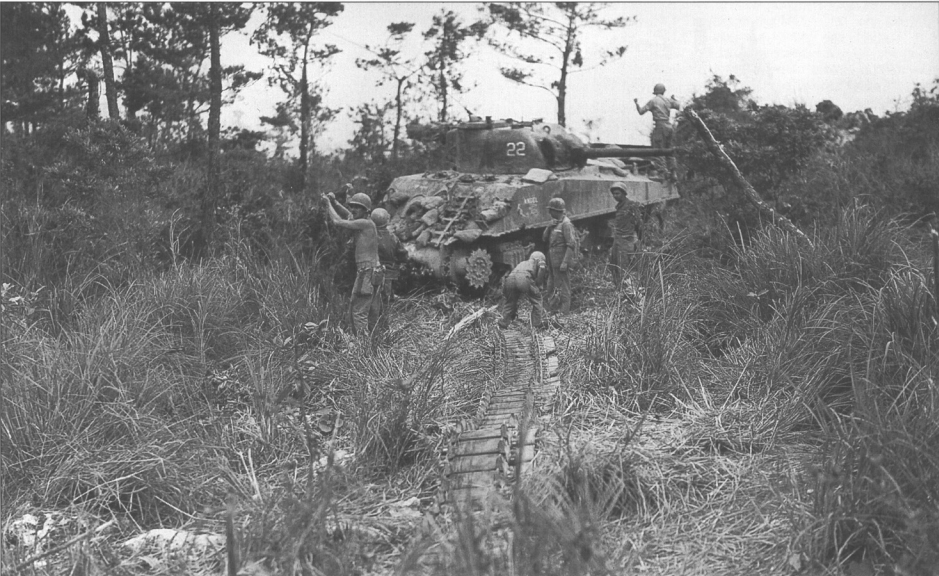
The crew of a M4A3 (W) named "Angel" of Co. A, 711th Tank Battalion hurriedly repair a thrown track while under Japanese sniper fire during fighting near Nakaza on Okinawa on 16 June 1945. Note that the track is fitted with extenders to lower ground pressure.
